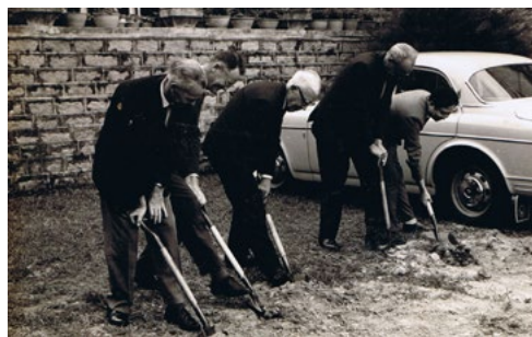
Ground breaking ceremony of HKAH-SR 香港港安動土儀式
